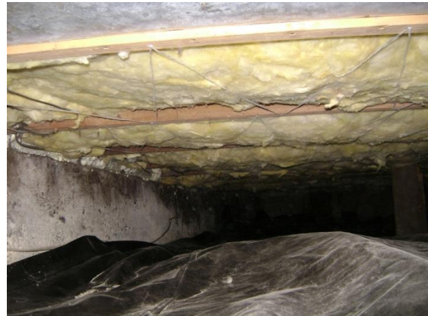
Home Crawlspace After
