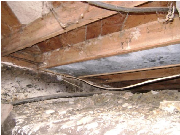
Home Crawlspace Before
